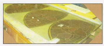
At right - A pattern for the construction of the window is created by placing craft paper and carbon paper atop the original stained glass panel and rubbing the impression onto the paper prior to disassembly. After the glass pieces are cleaned and set aside, they are reassembled along with any repair glass that may be needed. The lead channeling is cut and trimmed to hold all of the pieces of glass. The joining sections of lead are then soldered together.
